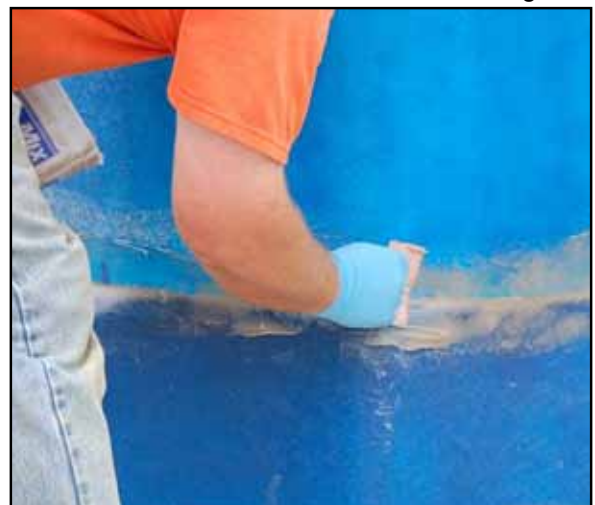
Figure 8: Applying Putty and Catalyst
