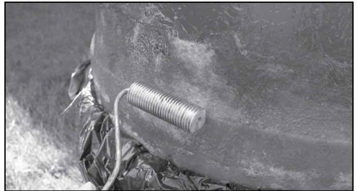
Figure 10: Remove Air Bubbles on Containment Sump
