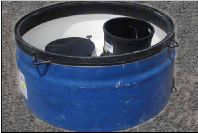
Figure 13: Sump backfilled
