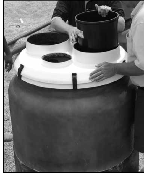
Figure 7: Aligning Multi-Port Sump Shield
