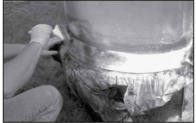
Figure 9: Apply Resin
