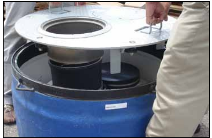
Figure 16: Installing Diamond Plate Cover
