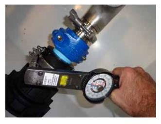
*Figure 5: Tighten Nut*6. Perform air test on the secondary layer of the XP pipe.
