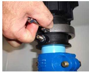
Figure 3: Install Test Clamp
